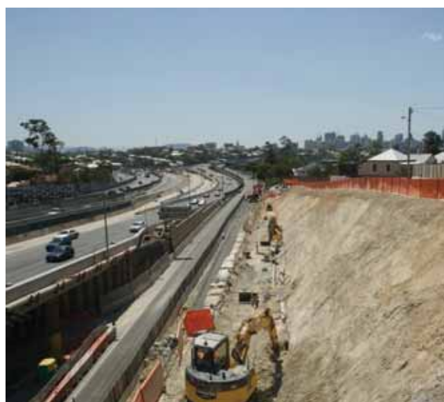
Batter slope under construction.
