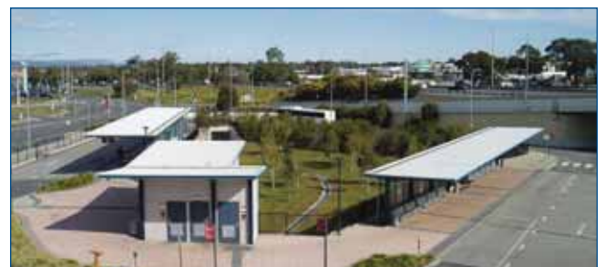
The existing bus and road infrastructure at Springwood.
